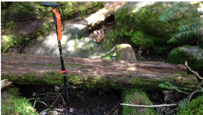
A repair project for 2017: a broken bog bridge on the Short Line. Chris Campbell photo.
