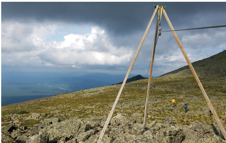
Alpine rigging near Thunderstorm Junction, during the crew's work on the Gulfside Trail in 2021. Sam Marshall photo.
