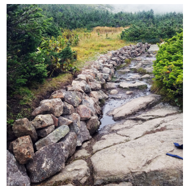
Above, Joey Schilke sawing lumber for the Diagonal; Reuben Morris and Julia Rudlaff replacing end-of-life bog bridges nearby; a new stone stair further down the trail, and the staircase on Starr King. Below left, field assessment of the Gulfside on a dry day in 2019, and at right in 2022 with its new screewall and water running in the trail (from Peabody Spring) as it usually does. The bottom photos show the crew moving a large “step rock” into place, to encourage hikers to stay on the trail and out of the alpine vegetation. Photos by Sam Marshall, Josie Bourne.
