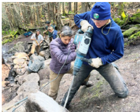
Left, the crew's field-built rigging system transports a rock up the slab surface; Max Buttrill photo. Center, Maya Barnett supports Annalise Brinks while she operates the rock drill. Right, closeup of drilling a hole for through-pinning. Emma Brinks photos.
