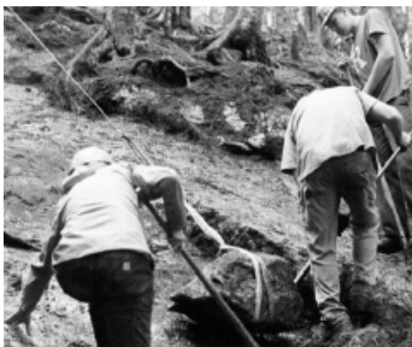
Left, the crew's field-built rigging system transports a rock up the slab surface; Max Buttrill photo. Center, Maya Barnett supports Annalise Brinks while she operates the rock drill. Right, closeup of drilling a hole for through-pinning. Emma Brinks photos.
